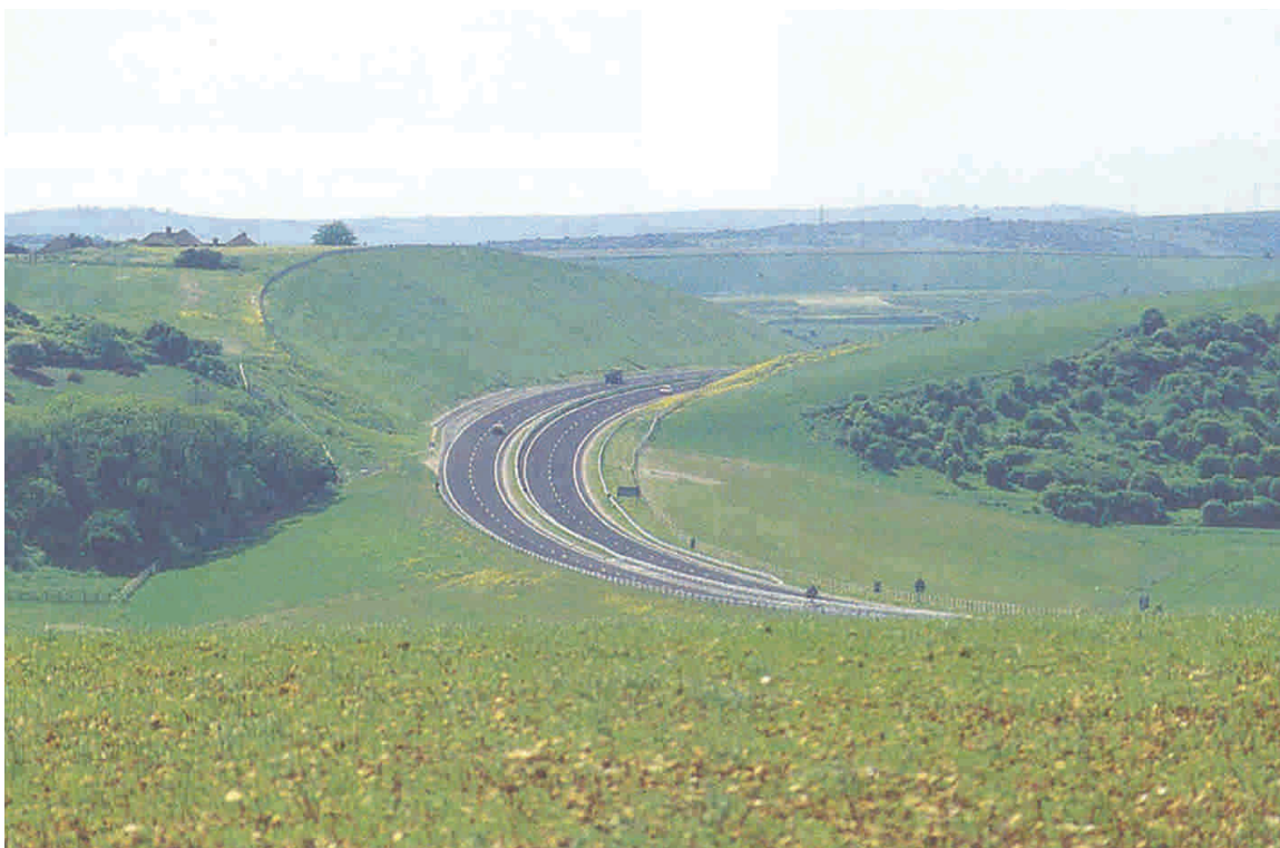
Figure 6.2 - The A27 Brighton bypass runs through the edge of the South Downs AONB in Southern England. Grading the cuttings and embankments to 1:6 fits the road into the downland character. (Photo by Highways Agency, UK)
