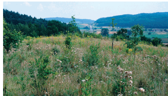
Figure 7.12 - On the landscape bridge Weiherholz in Germany (B31neu, 80 m wide) only the bushes were planted. Otherwise spontaneous growth of herbs and grasses was allowed, which was later managed by mowing. (Photo by V. Keller)
