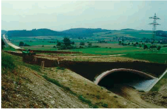
Figure 7.20 - The shape of the 80 m wide landscape bridge Hirschweg (B31neu, southern Germany) takes up the slope of the hill and leads animals across the road, which has been placed in a cutting. The picture was taken before the bushes planted as screens had grown. Nevertheless the overpass was intensively used by mammals as soon as it was covered with earth. (Photo by V. Keller)
