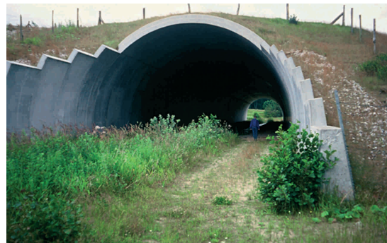
Figure 7.49 - This underpass in Denmark has a diameter of 13 m with 8 m clearance, and is 87.5 m long (at the top), 115 m (at the bottom). It is regularly used by fox, badger, marten, stoat and polecat - as well as by humans and horses. For ungulates the openness index would be too small. For underpasses under motorways the layer of soil above the overpass should be thicker to reduce noise inside the underpass. (Photo by B. Wandall)
