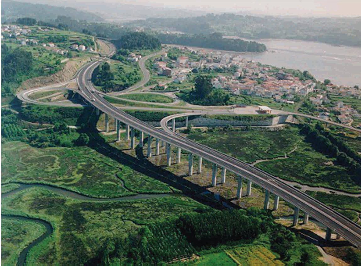
Figure 6.4 - Viaducts minimise landtake and fragmentation within a valley by allowing watercourses and any existing nature conservation interests to continue under the structure. This viaduct carries the A9 highway over an important wetland surrounding the River Mino (Galicia, Northwest Spain). (Photo by AUDASA, Spain)
