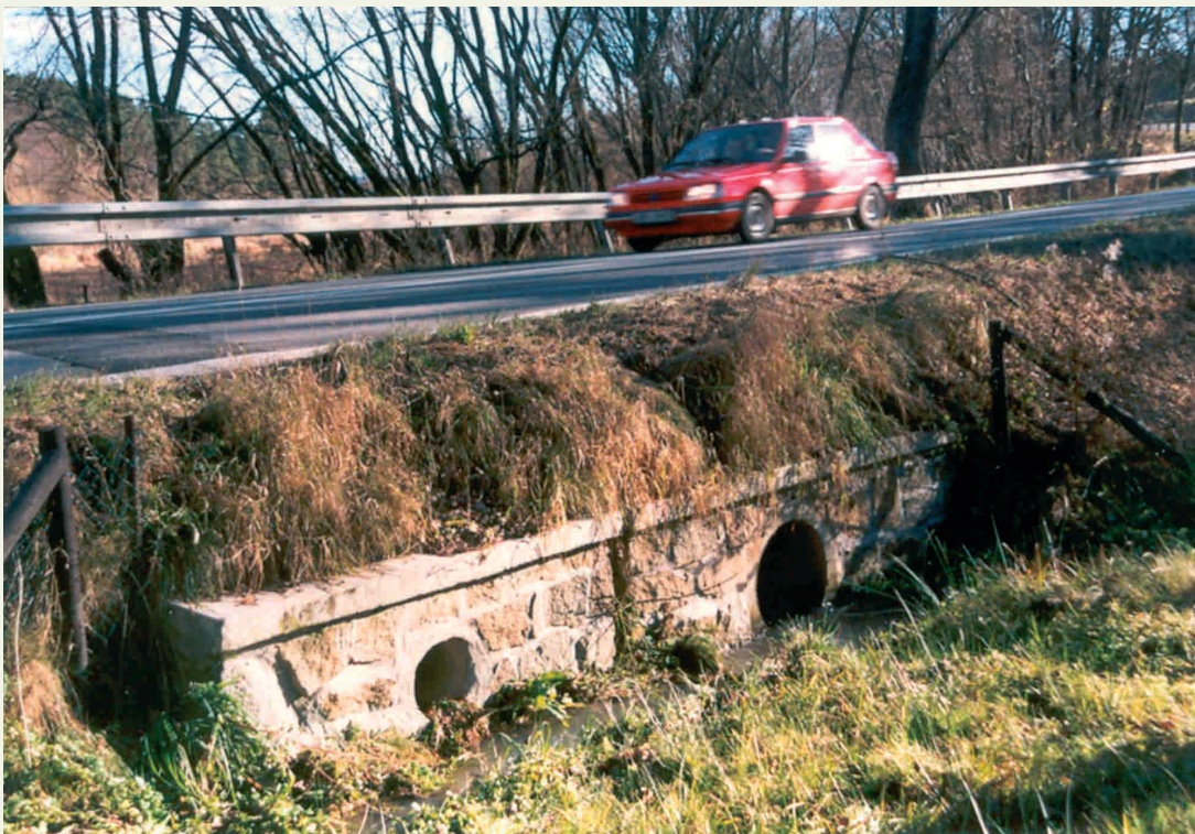
Figure 7.58 - Otters don't like to use water-filled culverts without dry parts. Small pipes placed above normal water level parallel to culverts, such as these ones crossing under a main road in southern Czechia, are used regularly. (Photo by V. Hlaváč)
