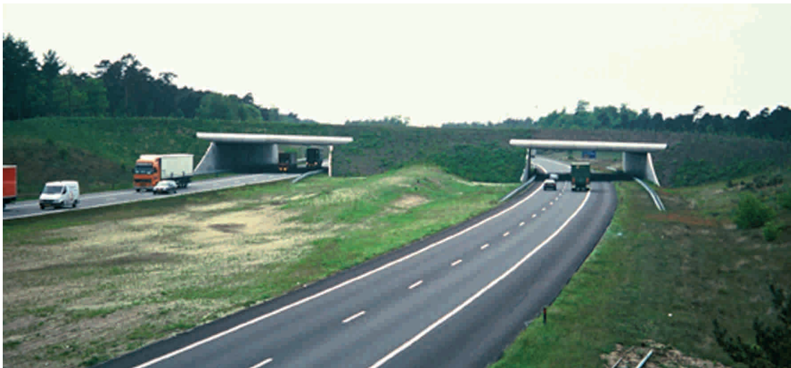
Figure 7.18 - The wildlife overpass Harm van der Veen (Kootwijk, the Netherlands) was built in 1998 over two separate parts of the motorway A1. This was a significant milestone, because it was the first overpass in the Netherlands to be built across an existing motorway. (Photo by H. Bekker)
