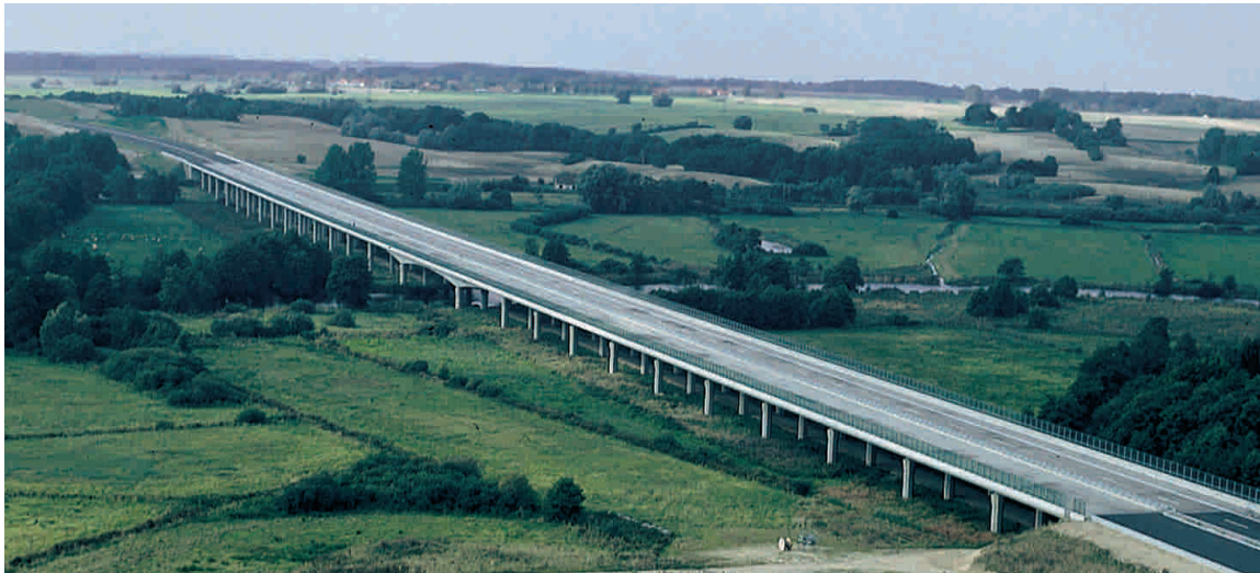
Figure 7.36 - Instead of building an embankment, the motorway A20 in northern Germany was built on pillars. This low viaduct preserves the floodplain and marshes below. (Photo by DEGES)
