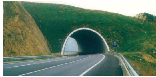
Figure 7.30 - A cut-and-cover tunnel in Spain improved for use by animals. (Photo by C. Rosell)
