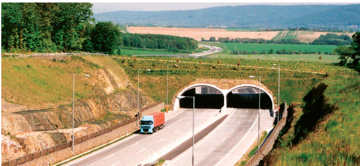
Figure 4.4 - Mitigation measures can be used to reduce the barrier effects of infrastructure. This is an overpass near Lipník nad Bečvou, Czech Republic, frequently used by a range of species including roe deer and wild boar. (Photo by V. Hlaváč)
