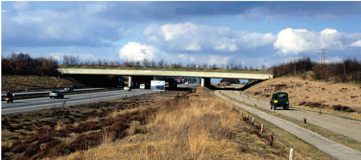
Figure 7.17 - The side view of Terlet north of Arnhem (the Netherlands) shows a straight concrete construction on pillars. The road level has been lowered to allow the overpass to cross at the level of the adjacent land. (Photo by V. Keller)
