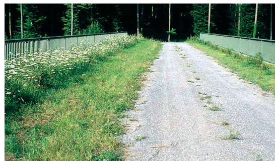
Figure 7.32 - A vegetated strip alongside a forestry track can enhance the permeability of infrastructure for small animals. A bridge across the high-speed railway line near Oberderdingen in Germany. (Photo by B. Georgii)
