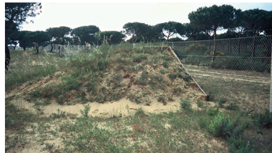
Figure 7.82 - An exit in the same area in the south of Spain designed for different animal species (Photo by H. Bekker)
