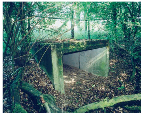
Figure 7.53 - A rectangular underpass for small animals, (1.2 m wide, 0.8 m high and 40 m long; A50 near Hernen, the Netherlands). This underpass is often used by badgers. (Photo by H. Cormont)
