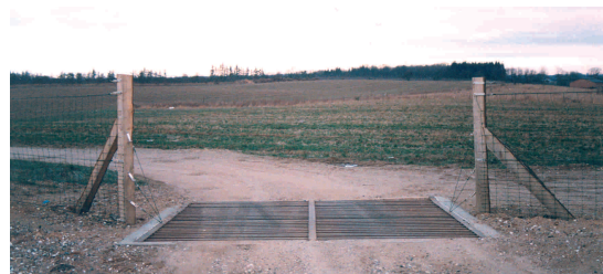
Figure 7.84 - Cattle grids are usually used on agricultural tracks as in this example from Denmark. However, they can also be used where a side road enters a main road. (Photo by B. Wandall)
