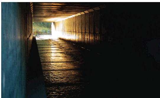
Figure 7.67 - Baffles in a fish passage in Norway during and after construction. (Photos by B. Iuell)
