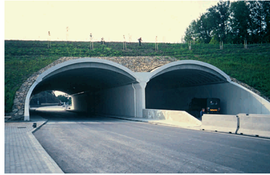
Figure 7.21 - Wildlife overpass in the Czech Republic with two prefabricated arches made of concrete. (Photo by H. Bekker)
