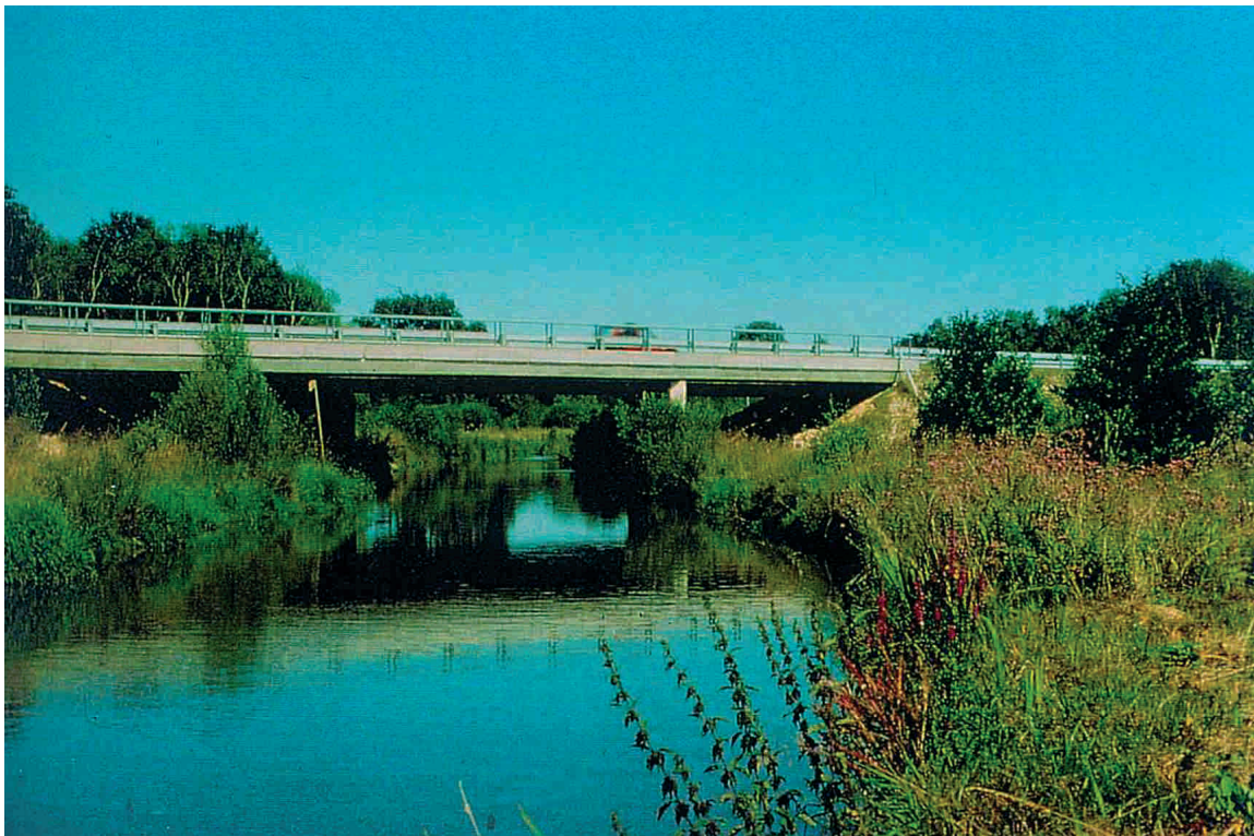
Figure 7.43 - A river crossing in France which preserves the natural river bed and has dry banks for movements by terrestrial animals. (Photo by J. Carsignol)
