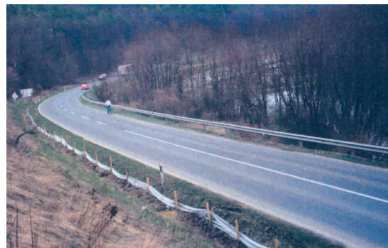
Figure 7.70 - A strong opaque plastic foil can be put up without stabilising wire mesh, as in this example from Hungary. However, the posts should not be placed on the side the amphibians approach from to improve the guiding function of the fence. (Photo by M. Puky)
