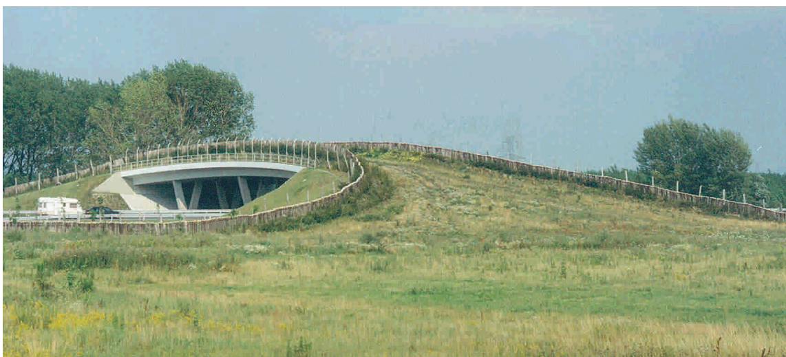
Figure 7.15 - In this example from Hungary the motorway was not cut into the surroundings. The access had therefore to be levelled out. The fences guide animals along the road verges to the overpass. (Photo by P. Farkas)
