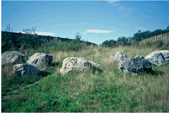
Figure 7.28 - Boulders were placed on this overpass on highway 64 in France to block access for cars. (Photo by H. Bekker)
