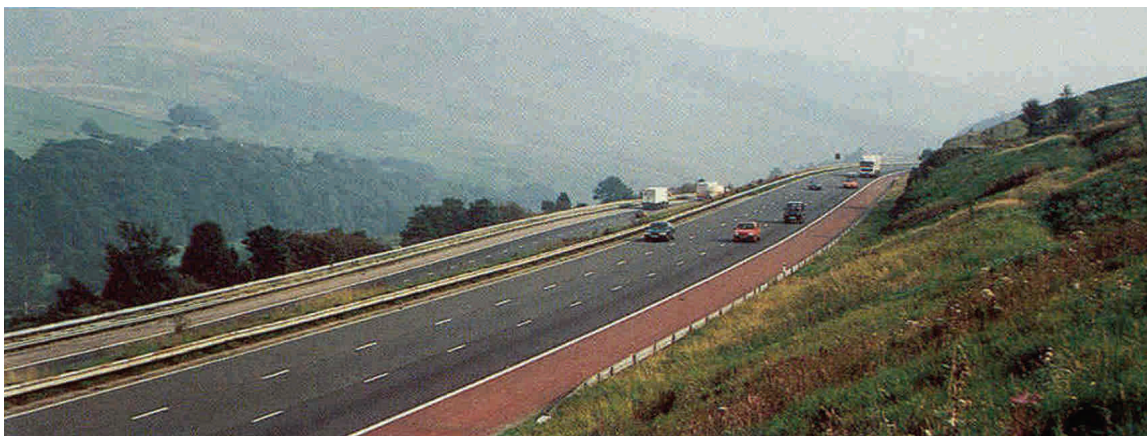
Figure 6.3 - M6, Cumbria in Northern England. The road follows a major ridge and avoids the river valley. Verges are restored to the classic upland vegetation types. (Photo by Highways Agency, UK)
