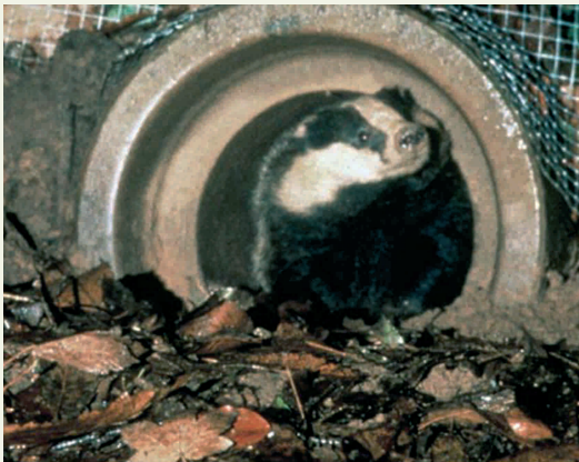
Figure 7.56 - A small fauna underpass in the Netherlands with a badger. This kind of tunnel may be used by small carnivores, mice and amphibians (Diameter: 0.3-0.6 m, length: 5-60 m). (Photo by Vereniging 'Das en Boom')
