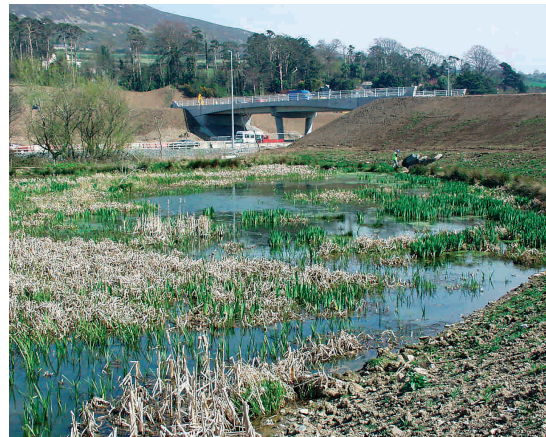
Figure 8.3 – Example of wetland construction in the Glen of the Downs, Ireland. Above: during construction, below: on completion. (Photo by R. Nairn)
