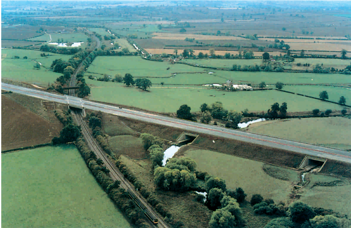
Figure 6.5 - M40, Cherwell Valley, Oxfordshire. The embankment is a dominant feature but care has been taken to retain the character and form of the river on both sides of the road. (Photo by Highways Agency, UK)
