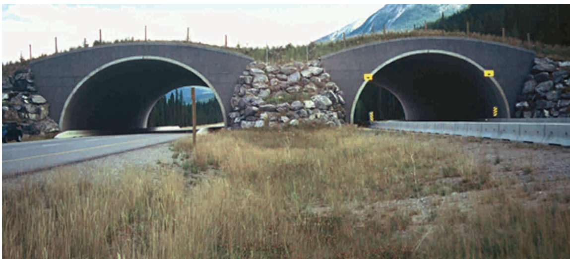
Figure 7.19 - This wildlife overpass in Banff national park on the Trans Canada Highway was built with prefabricated elements across an existing road. (Photo by H. Bekker)
