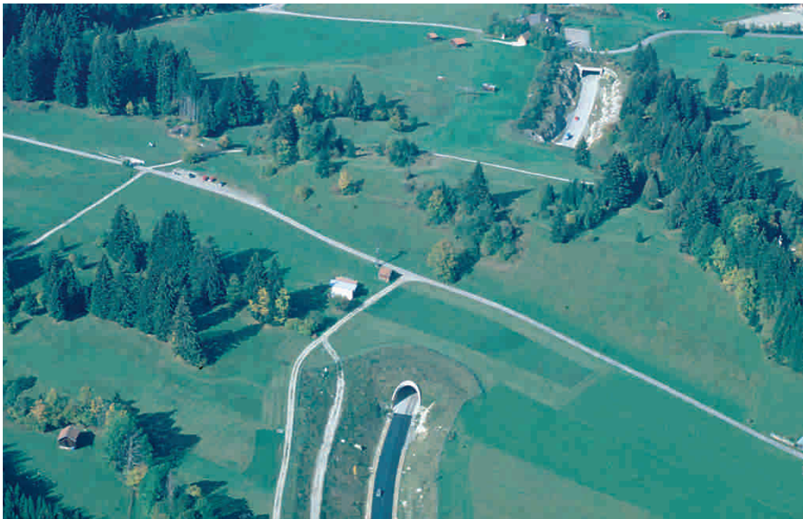
Figure 6.9 - Bored tunnels leave the habitat above intact. They are particularly suitable in hilly areas like this example from Bavaria, Germany. (Photo by B. Georgii)
